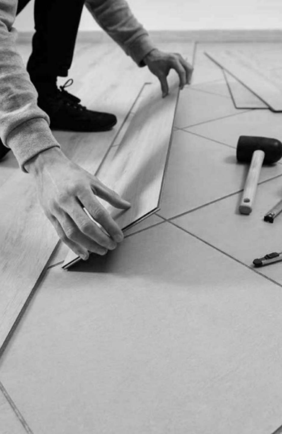
Installation is fast and easy thanks to the unique click lock system. Click Lock Technology works perfectly for both the long and short sides of the flooring panel and ensures there are no unwanted gaps or spaces between floorboards.
